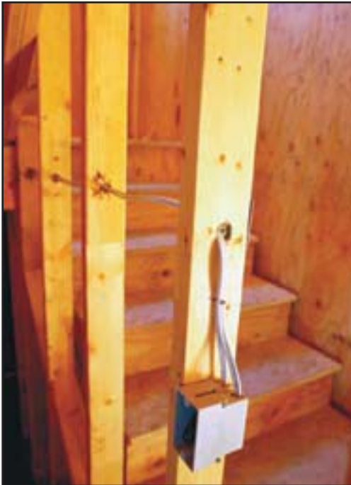
Nonmetallic sheathing helps protect wires from damage.
