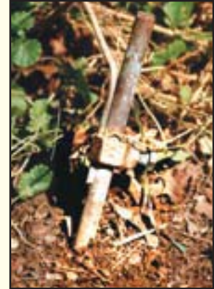
Grounding rod in the earth.
