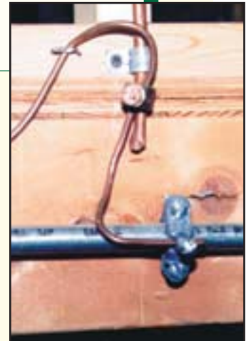
Install bonding jumpers around nonconductive material.
